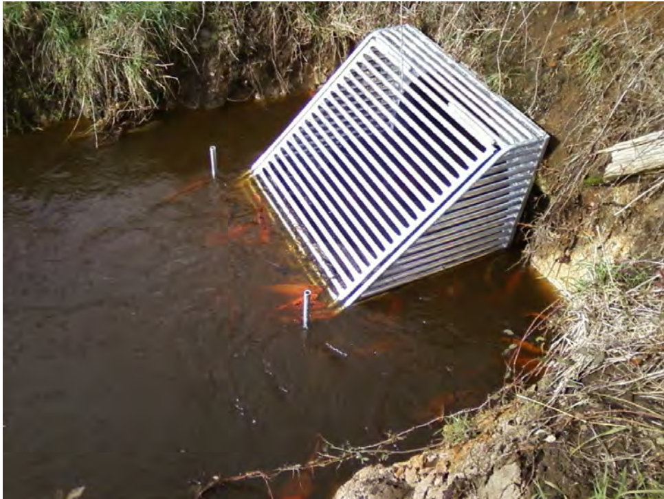
Figure 2. Permanent fish barrier installed on downstream side of road culvert outlet to Lake Ohinewai showing around 60 adult koi carp attempting to pass the barrier.
