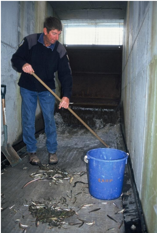
Figures 5 and 6: Cleaning internal fine mesh screens, placed horizontally to assist gravity driven filtration and a section view showing flow through screen.
