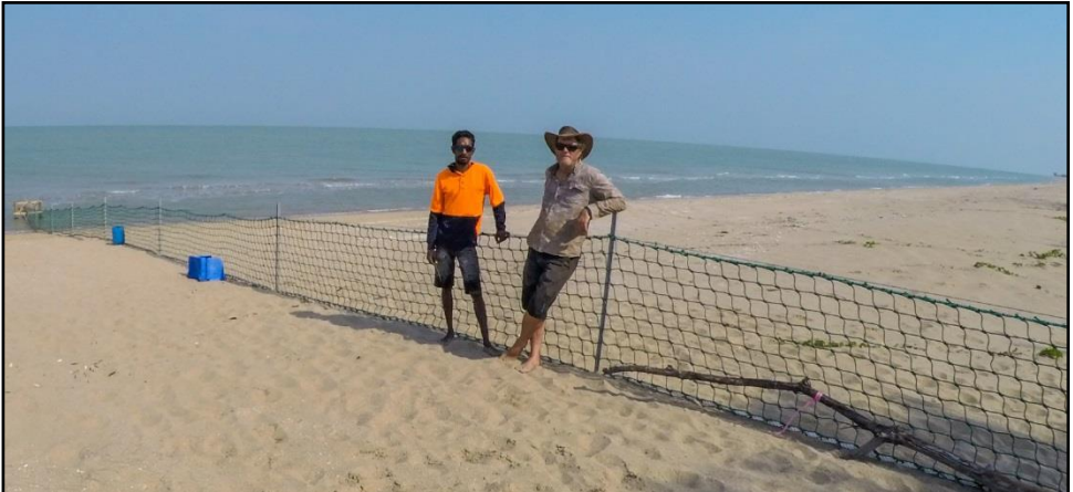
APN Cape York ranger staff and the completed spit fence (one of two), protecting 10 km of turtle nesting habitat from potential pig predation. The fence is mostly wire (as in the exclusion fencing section) but has netting on the beach.
