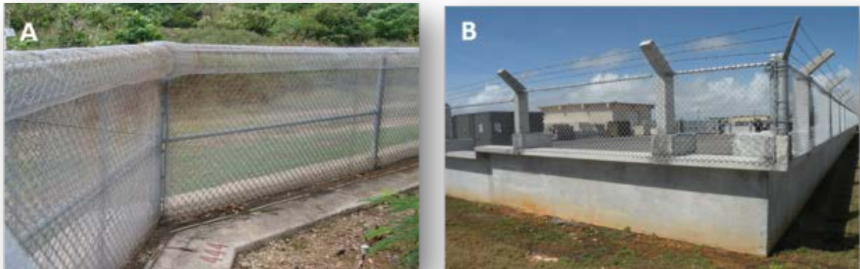
Figure 2. Examples of permanent barriers A) hardware cloth bulge barrier, B) hybrid concrete barrier with security fence above.
