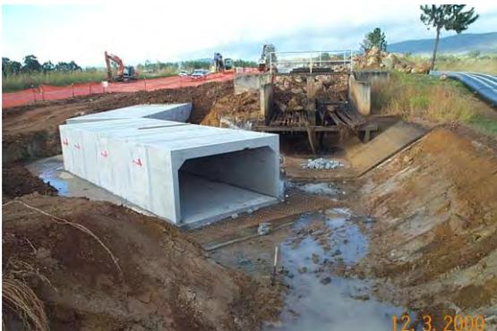
**Figure 6:** Construction of box culvert outlet.
