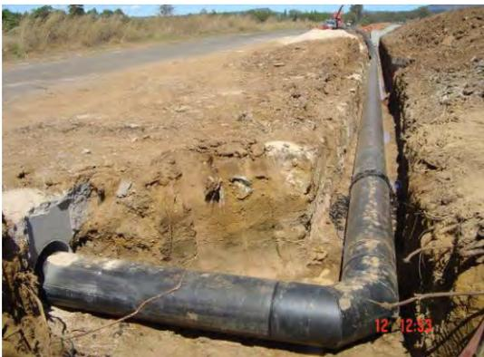
**Figure 8:** Filtrate pipeline from fish screen at road crossing.
