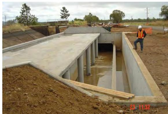
**Figure 7:** Completed concrete screen structure before screens installed.
